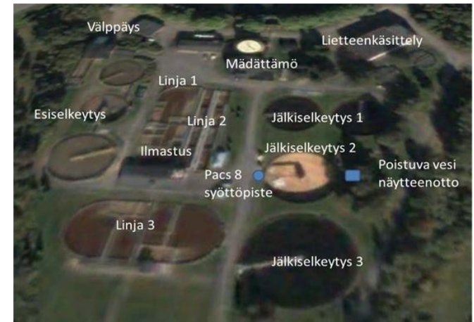
Overview of Mikkeli WWTP
